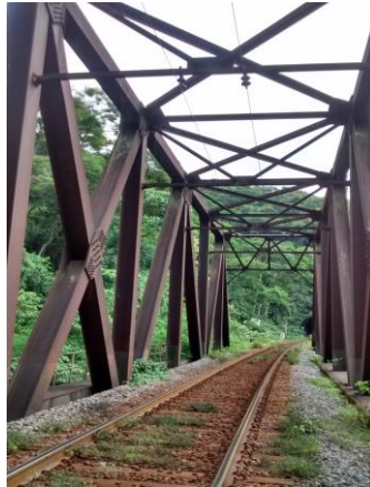
Figure 1 - Truss bridge over the Fumaça Waterfall
