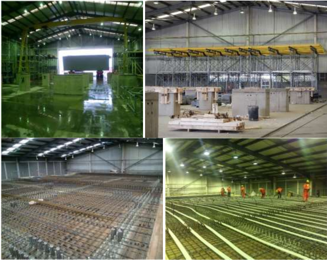
Figure 6 – Preparation of formwork for pre-casting the deck slab.
