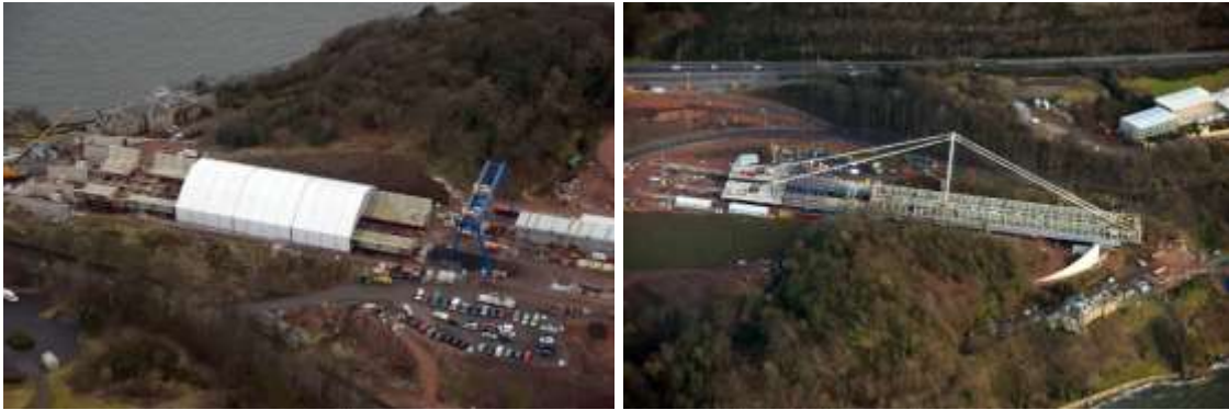
Figure 12 - North viaduct during assembly and launching.
