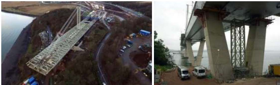
Figure 13 – North viaduct during assembly and launching.
