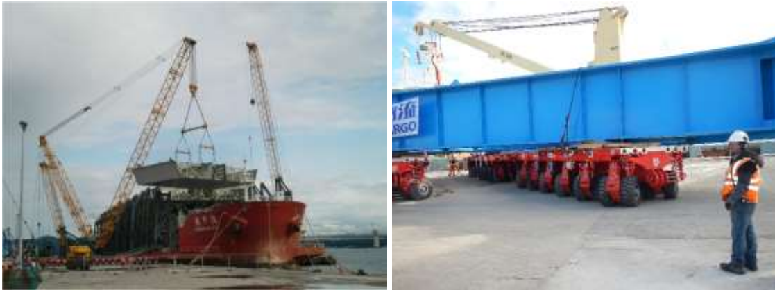
Figure 5 – Off-loading and yard transportation on SPMT's.
