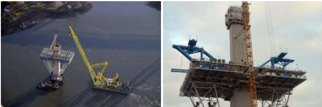
Figure 8 – Taklift 6 installed falsework, tower segments and erection gantries.
