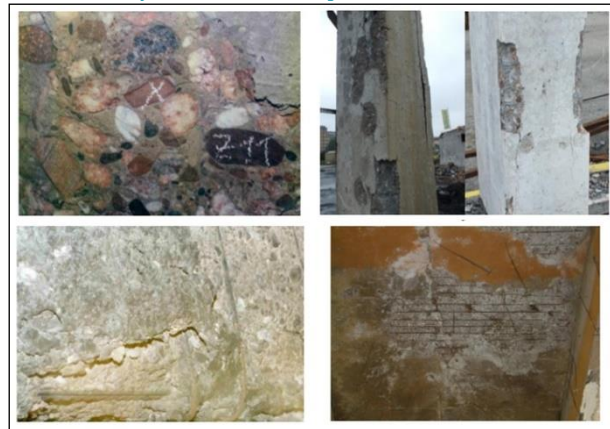
Figura 1 – Exemplos de Corner spalling, e sloughing off e aggregate spalling (MALESEV, RADONJANIN (1999), adaptado).
