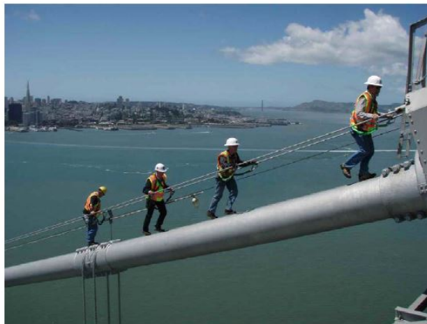
Figure 2.5.14 Handrail on Suspension Bridge
